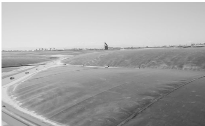
Seven-acre covered lagoon at Gallo Farms. Inclined screen solids-separator is visible in distance.
